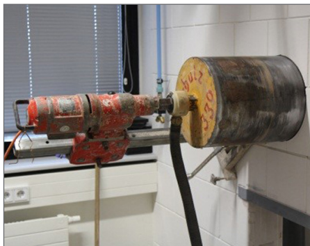
Fig. 2 – core hole drilling
