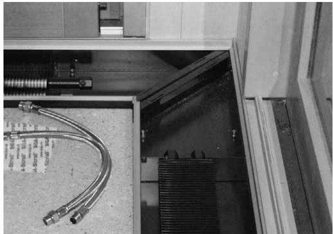
Example connection in series with flexible hose (included in delivery), 90° angled version on request
